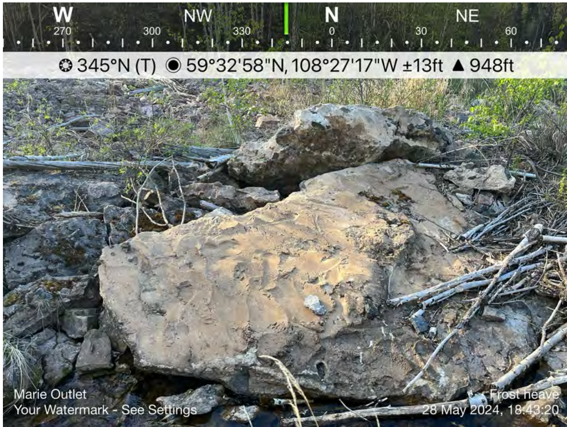
Photo A1 – Marie Reservoir Spillway ice jacked block near entrance inlet (May 2024)
