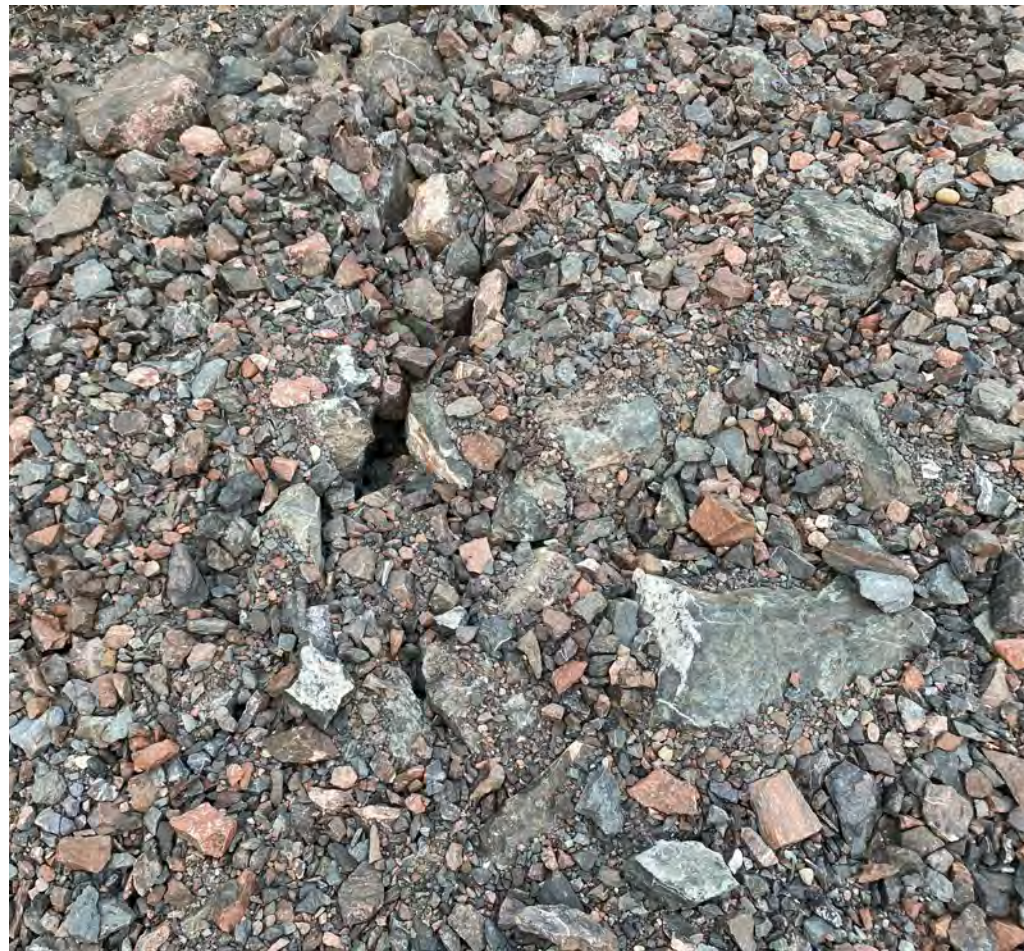
Photo D08—Settled fine material along bottom bench. Material is settling into voids in the underlying waste rock (July 2024)
