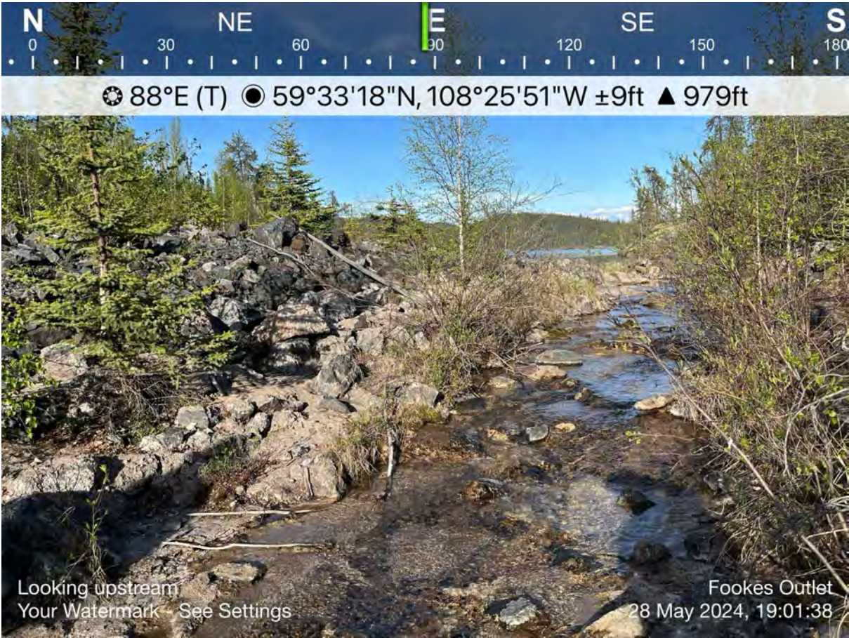
Photo B5 – Fookes Reservoir Spillway showing broken rip-rap on north side of channel.
