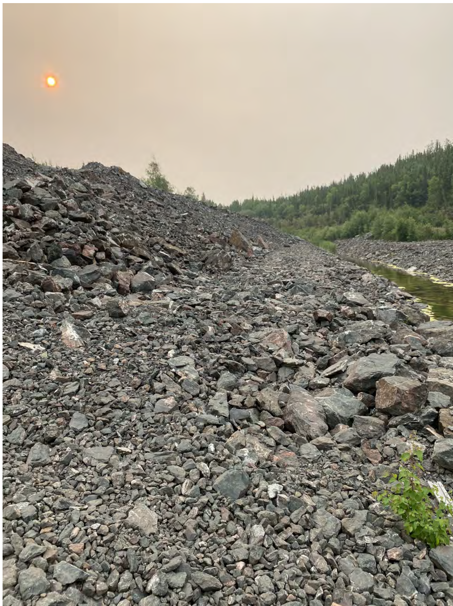
Photo D07—View of bottom bench with fine material covering waste rock to allow vehicular traffic during remediation (July 2024)
