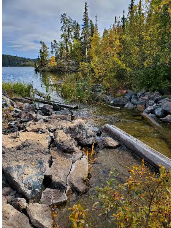
Photo 17: Looking upstream along the outlet spillway showing the ice-jacked slabs of grout-intruded rip-rap on the sides of the spillway. Photo taken on September 16, 2020.
