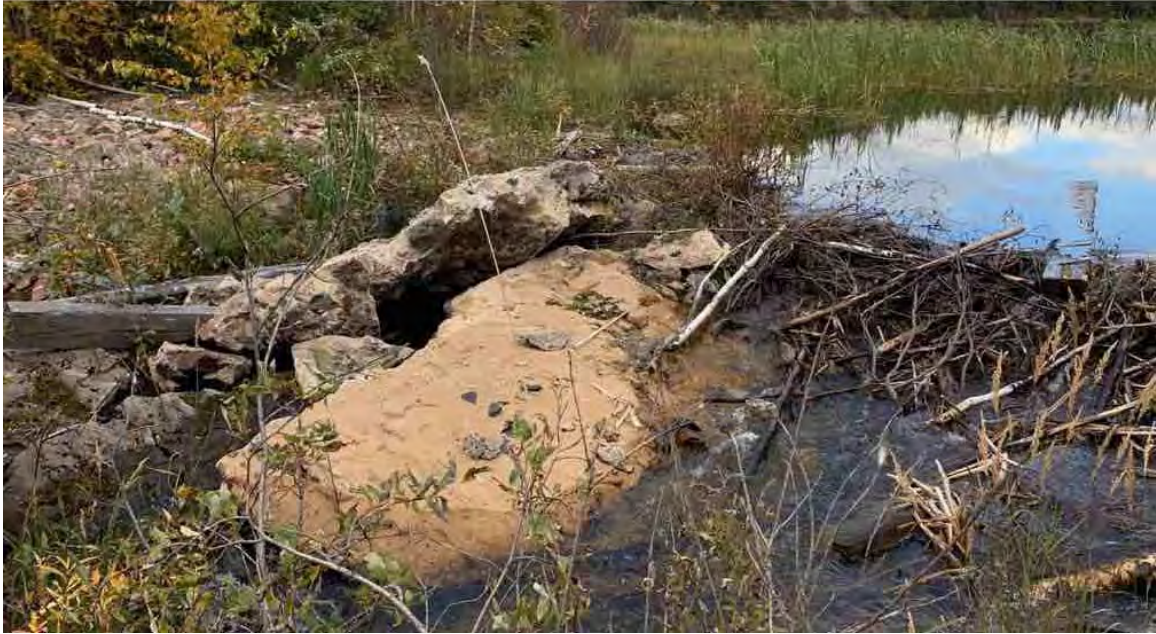
Photo 23: Looking at the ice-jacked slabs of grout-intruded rip-rap on the right side of the Marie Reservoir outlet spillway, near its upstream end on September 16, 2020. Beaver dam is visible immediately to the right of the slabs.
