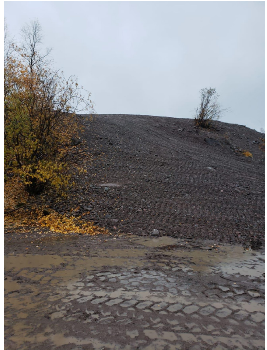
Photo 19: Final placement of the gravel cover layer.
