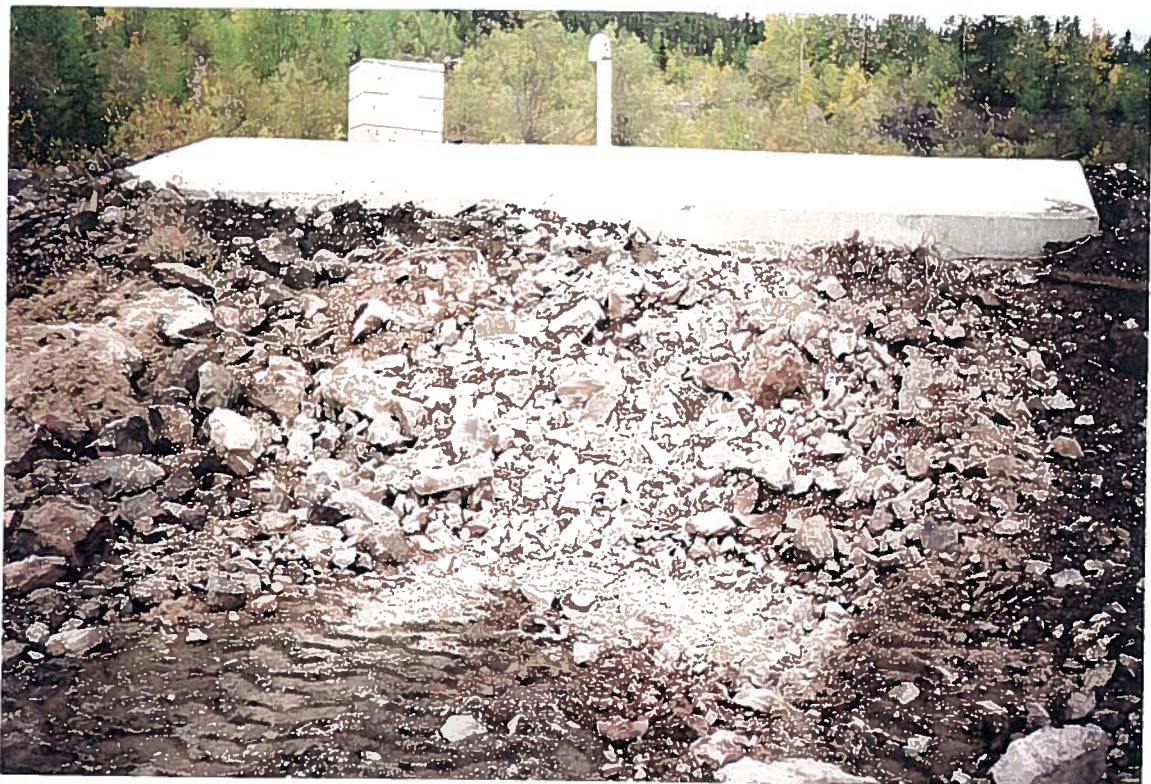
Photograph 8: Completed structure after placement of fill.
