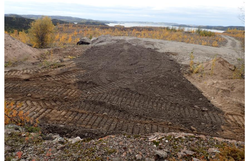
Photo 12: Looking southwest - Placement of waste rock (various sizes).
