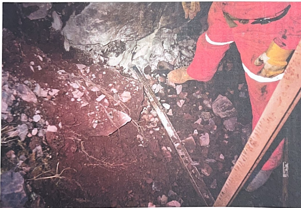
Photograph 2: Rock bolting and welding on the sides of the structure.
