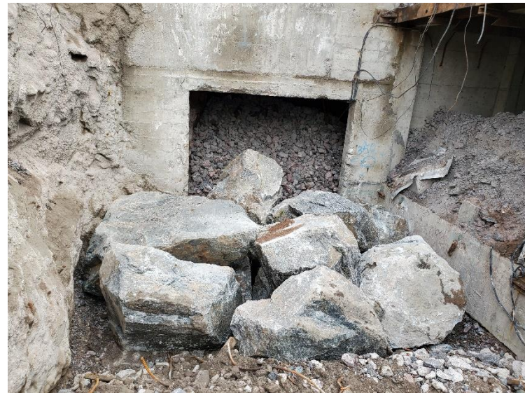
Photo 14: Total of 11 boulders placed for the permanent closure of Raise 2.
