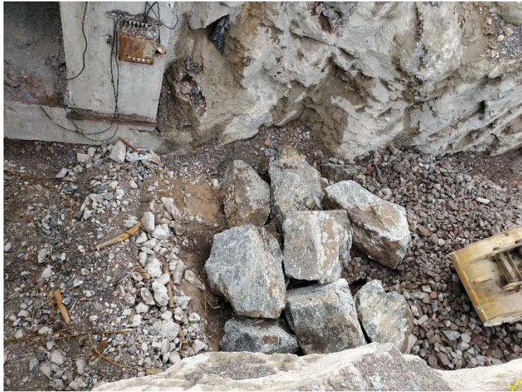
Photo 10: Top view of the 15 boulders placed at Raise 3.
