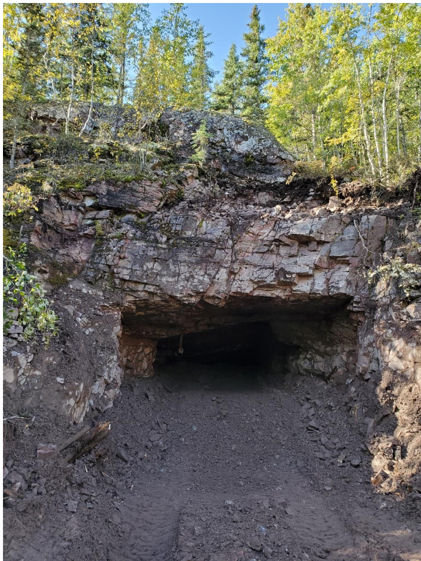
Photo 3: Stages of Backfill placed in the Fishhook Bay Adit
