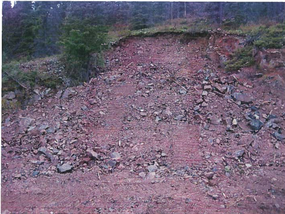
Figure 5 –Adit Following Closure Activities
