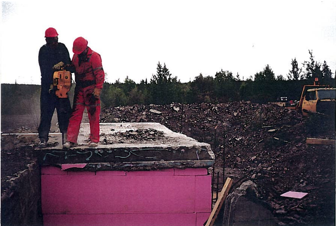
Photograph 2: Demolition of the existing ridge cap.
