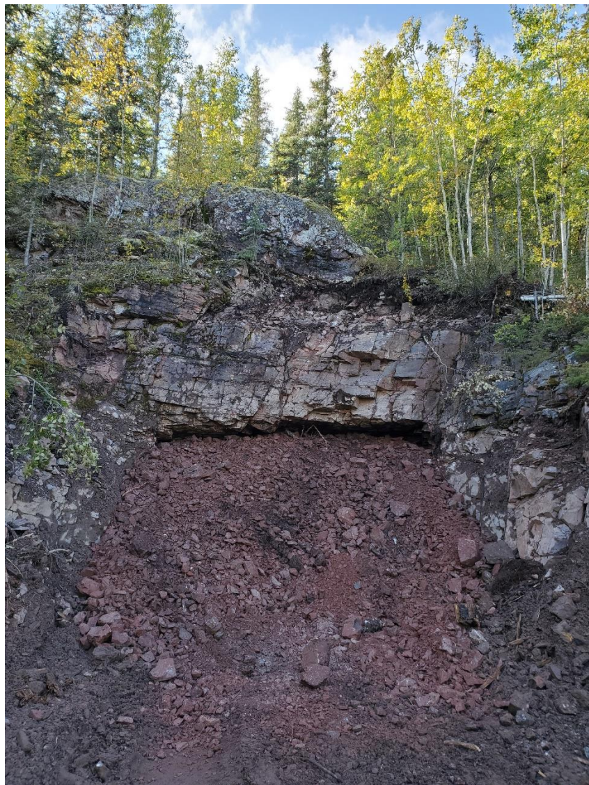
Photo 4: Stages of Backfill placed in the Fishhook Bay Adit
