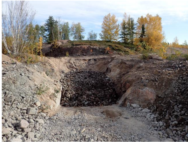
Photo 9: Placement of sorted waste rock, tight against the back (competent rock passing approximately 200 mm).
