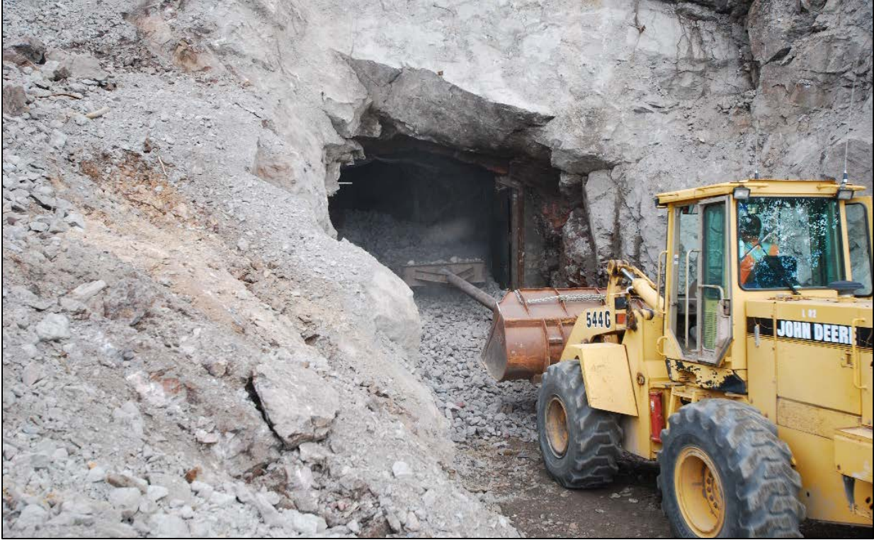
Figure 4: Backfilling Adit with Loader Attachment
