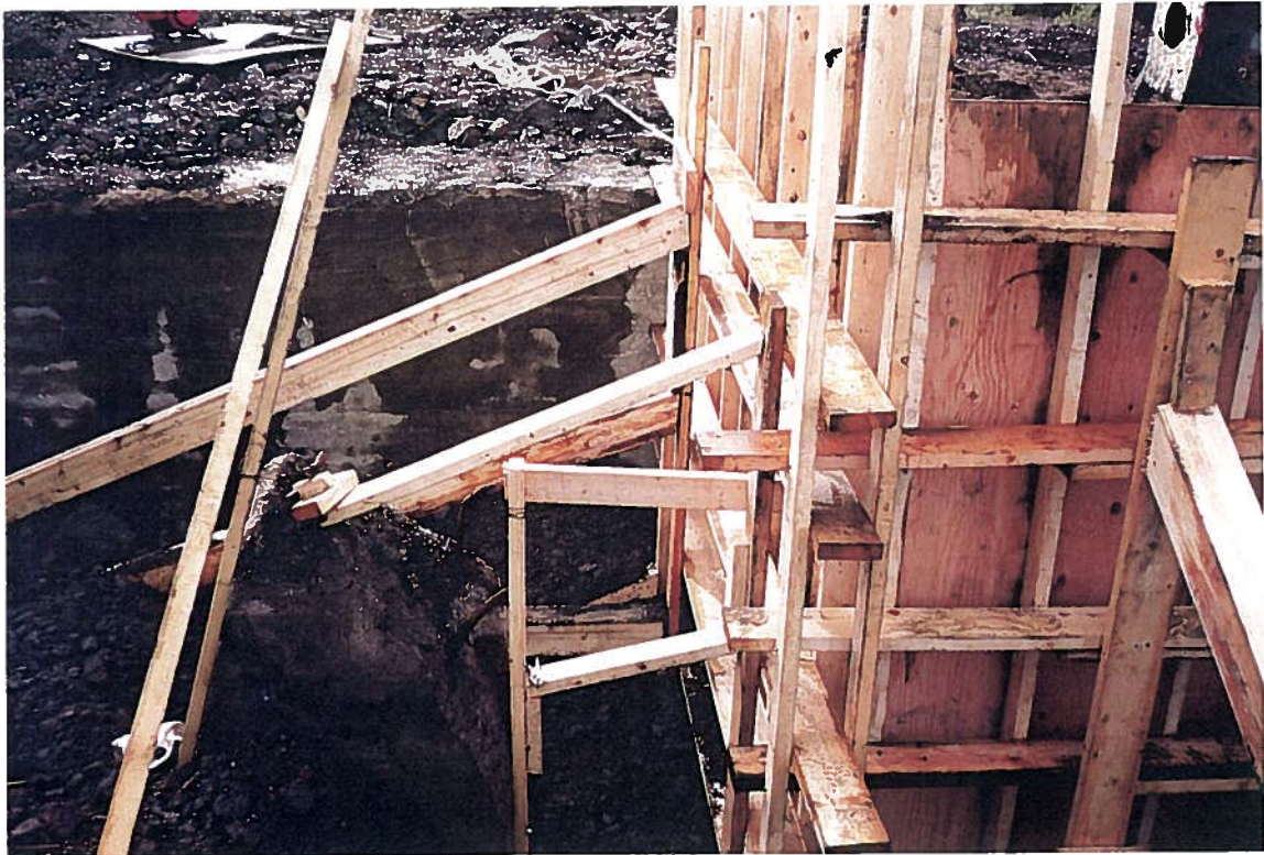
Photograph 4: Form work and false work on the walls.
