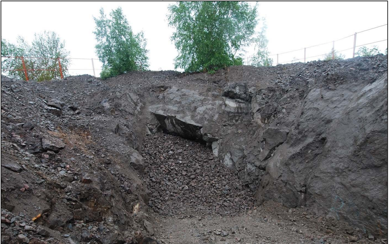
Figure 6: Backfilled Adit
