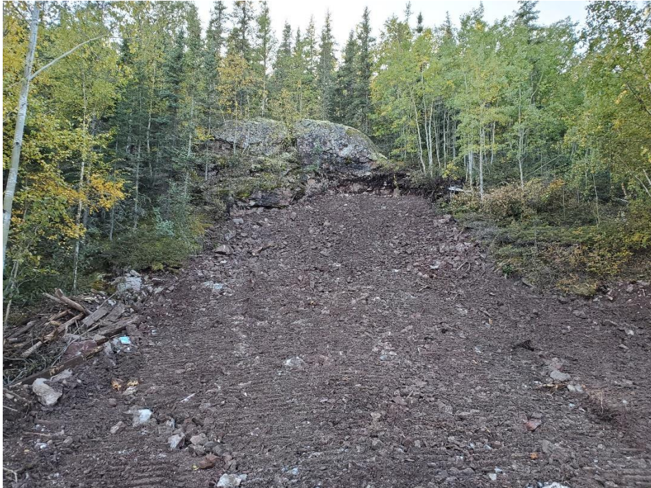
Photo 5: Final Placement of Backfill material along the Fishhook Bay Adit.
