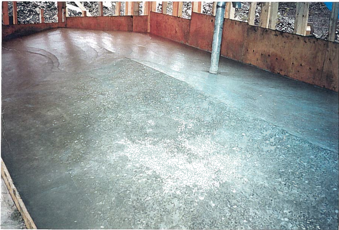
Photograph 6: Roof slab after the steel trowel finish.
