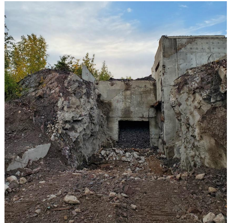
Photo 2: Overview of the Custom Crusher Raises Site.
