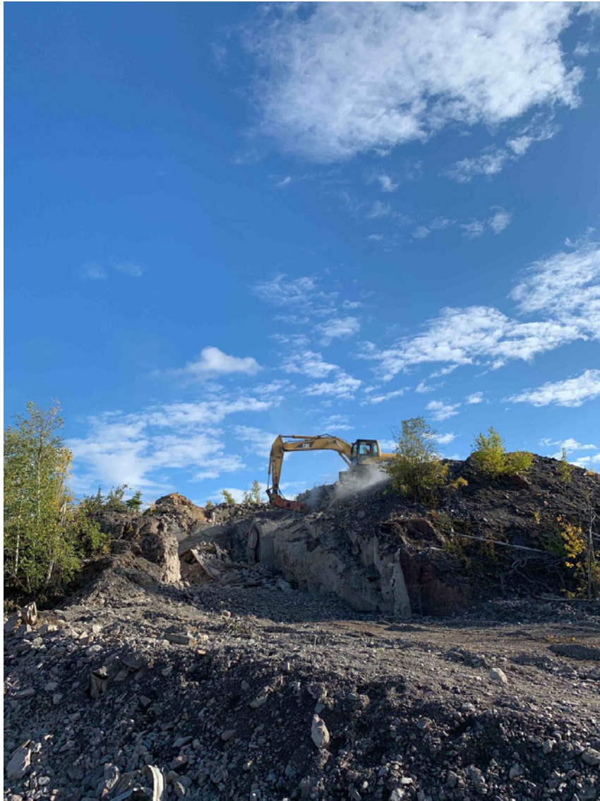
Photo 18: Demolition of the concrete dump chute.
