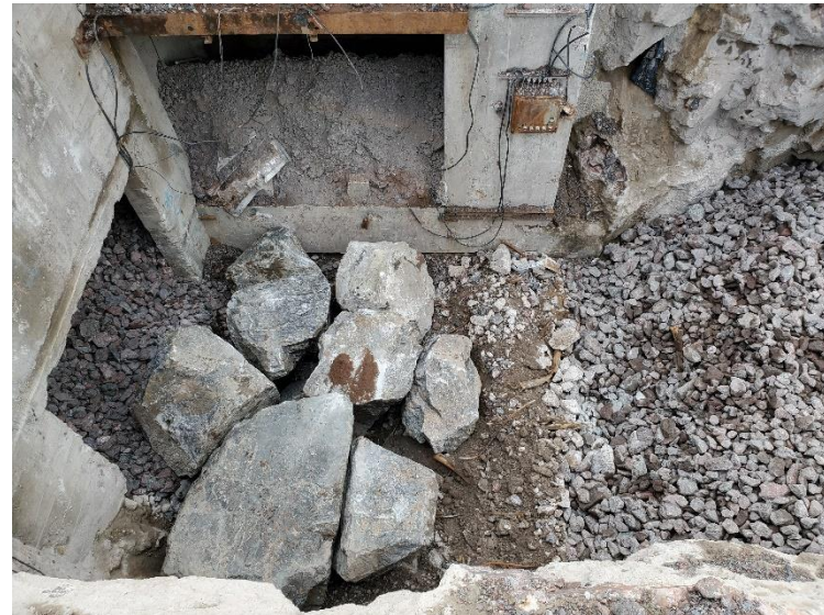
Photo 15: Top view of the 11 boulders placed at Raise 2.
