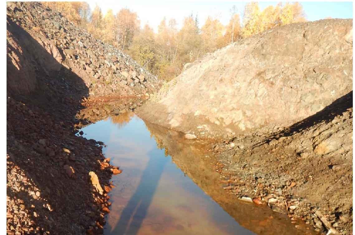
Photo 7: Looking West along channel base from approximately Station 0+270
