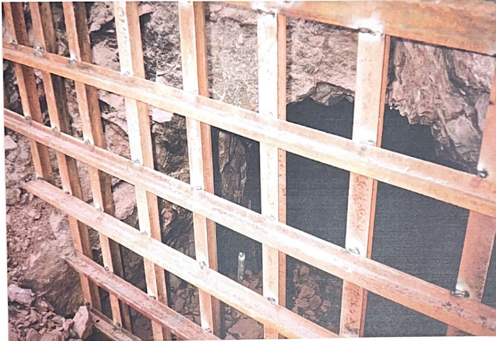
Photograph 5: View of welds at all cross members.
