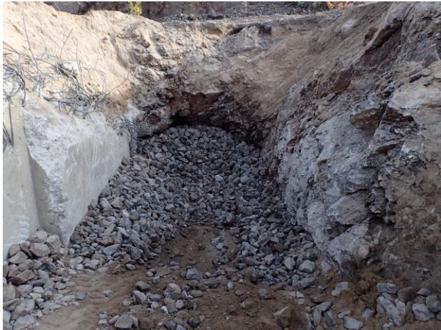
Photo 8: Placement of sorted waste rock (competent rock passing approximately 200 mm).
