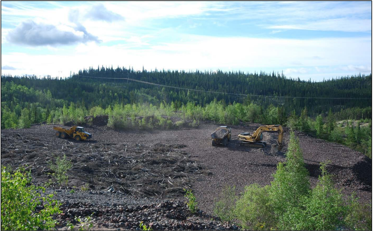
Figure 5: Sorted Waste Rock Used for Backfill Material
