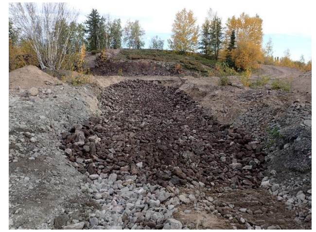
Photo 10: Placement of sorted waste rock over the brow (competent rock passing approximately 200 mm).
