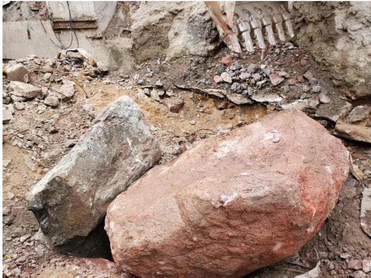
Photo 9: Rock Number 2 contributing to the wedging effect at Raise 3.
