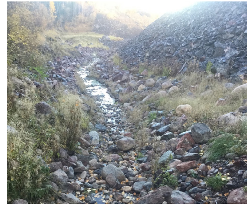
Photo 4: Looking West at Channel Base from Station 0+015 to Station 0+030
