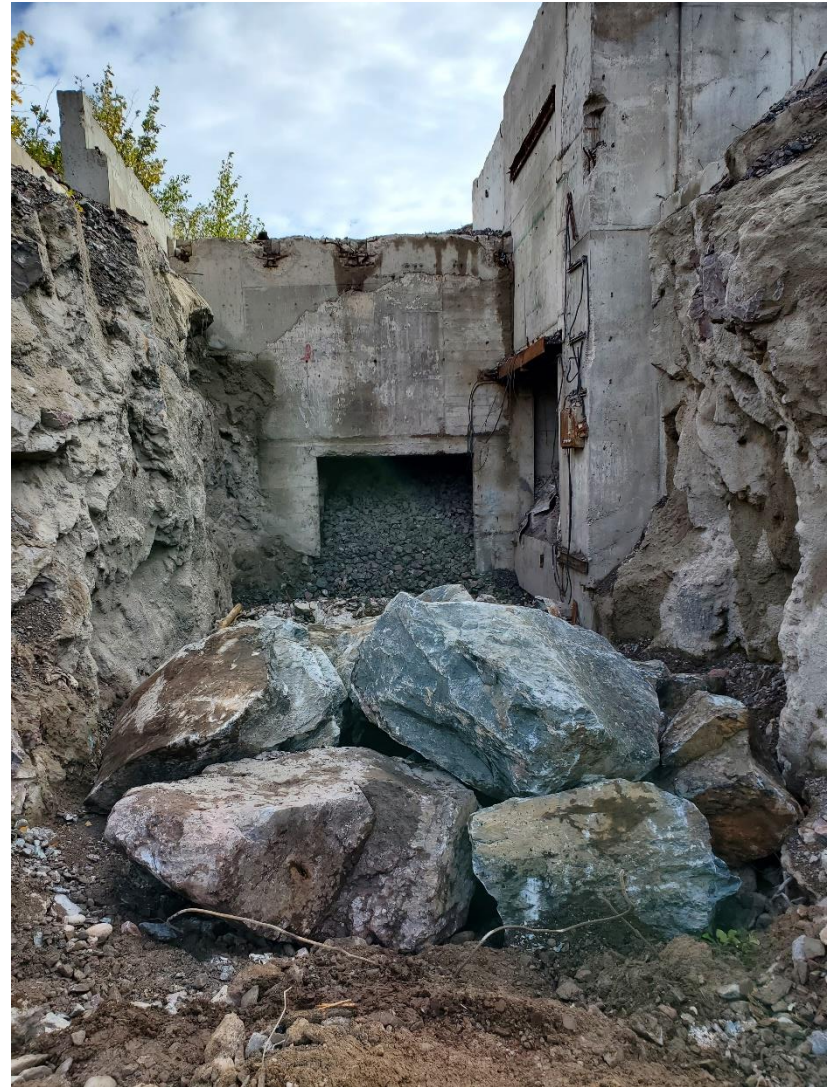
Photo 11: Total of 15 boulders placed for the permanent closure of Raise 3.
