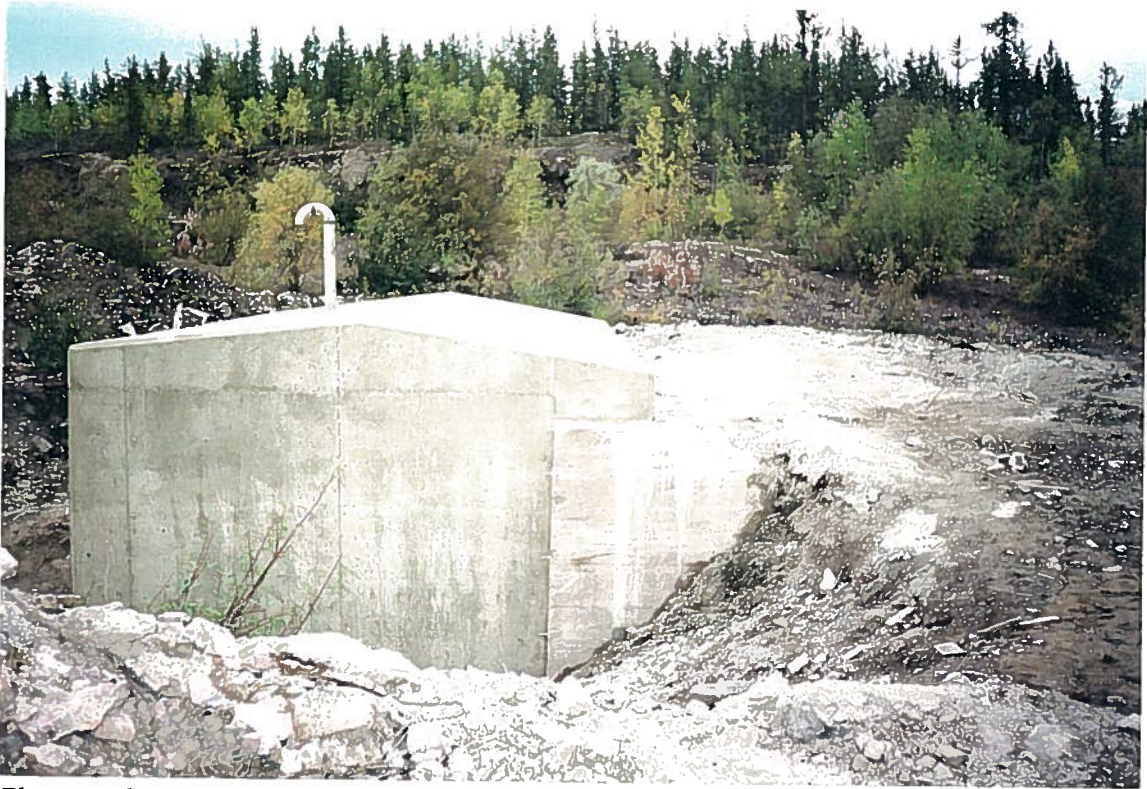
Photograph 7: Completed structure after the forms were removed.
