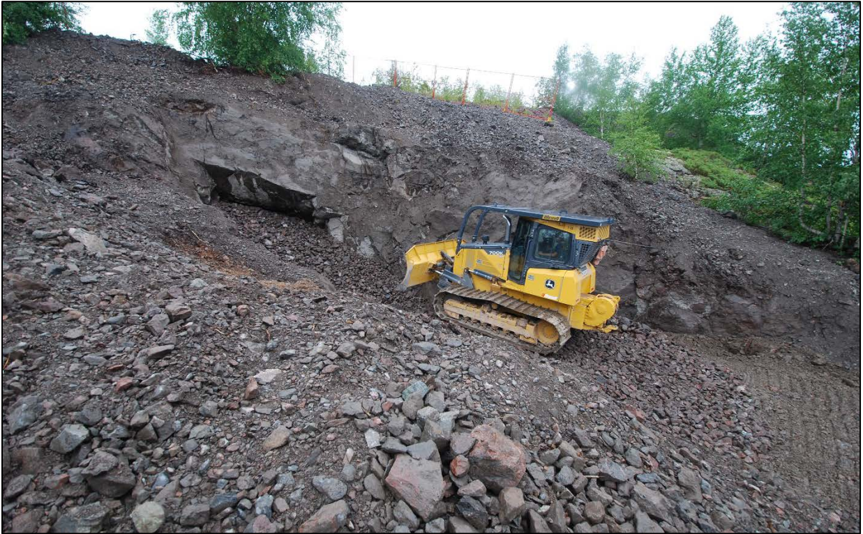
Figure 7: Placing Sorted Waste Rock in Adit Entrance
