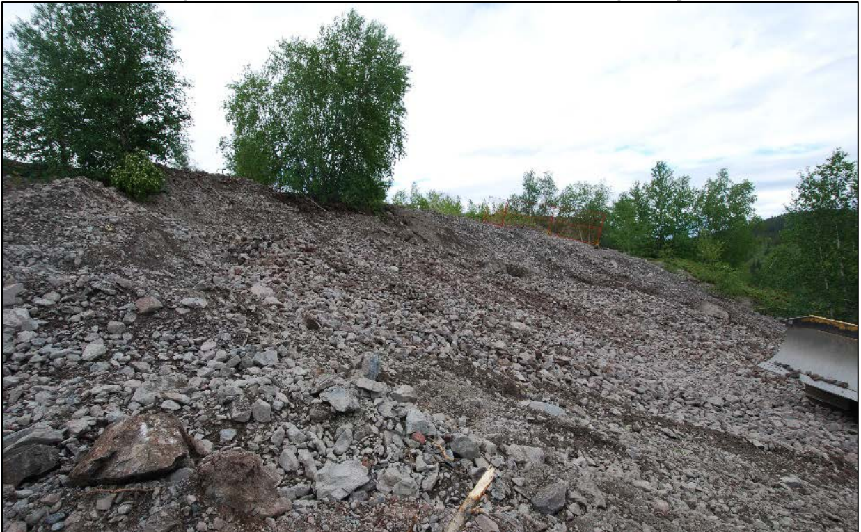
Figure 8: Backfilled Adit Entrance with Material Placed to Original Slope
