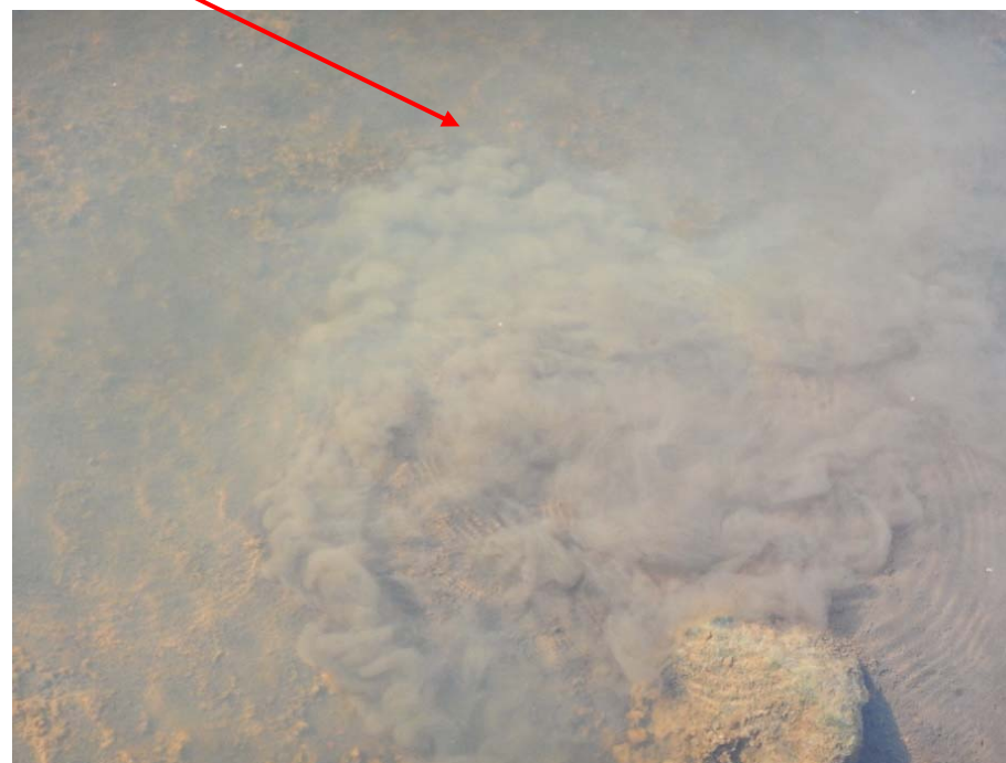
Photo 10: Looking South at Channel Base Sedimentation after resuspension (Station 0+215)
