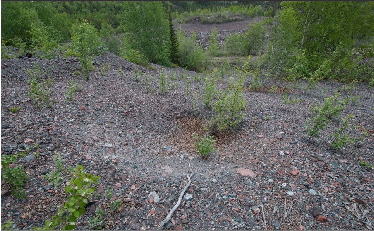
Figure 1: Subsidence Observed Above the Waste Haulage Adit
