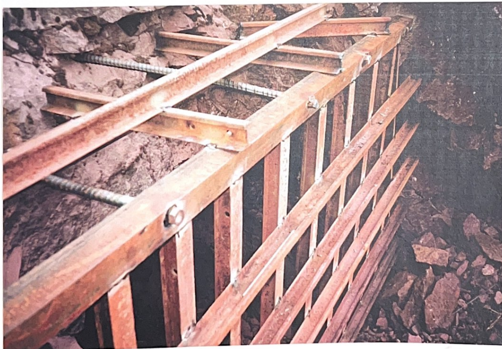
Photograph 4: Structure rock bolted and welded in place.
