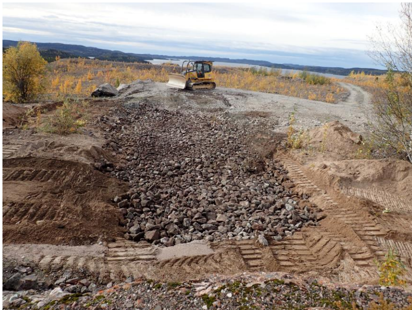
Photo 11: Looking southwest - Placement of sorted waste rock to level (competent rock passing approximately 200 mm).
