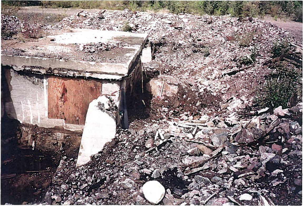
Photograph 1: Excavation around existing Eagle Mine shaft cap.
