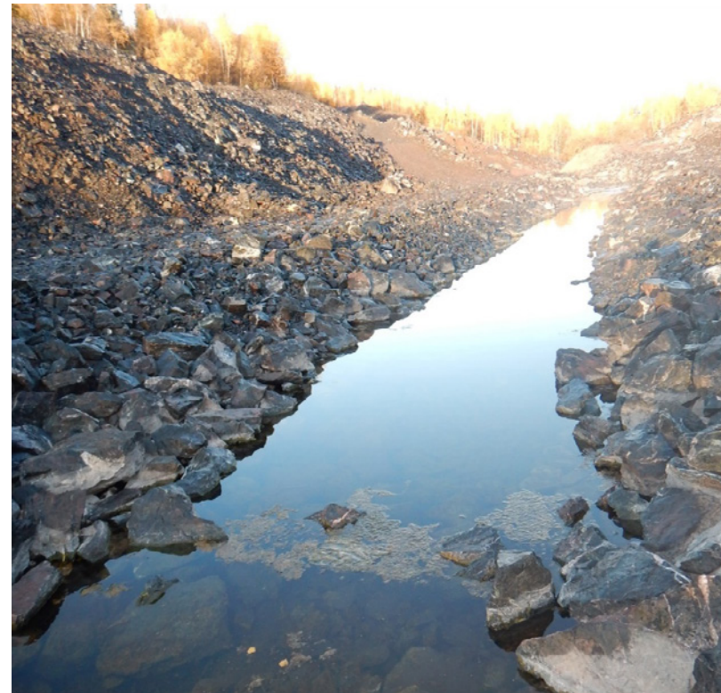
Photo 6: Looking West along channel base from approximately Station 0+135
