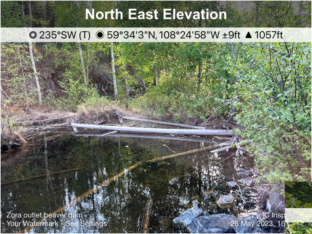
Photo E05—View of well-established beaver dam at the outlet of Zora Lake, looking downstream (May 2023)
