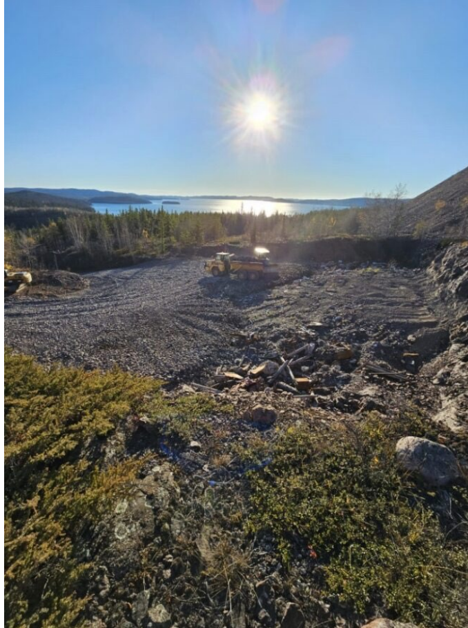
Photo 2- Lower Fay Pit being covered with waste rock
