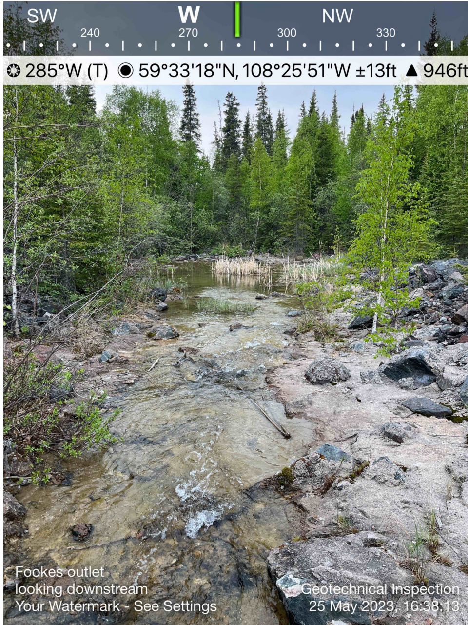
Photo B3 – Fookes Reservoir Spillway looking downstream (mid channel)
