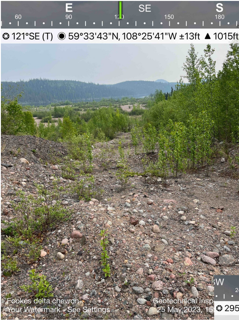
Photo C2 – no ponded water (May 2023). This area previously had ponded water on waste rock cover at bottom of hill near north access road during freshet in 2022.
