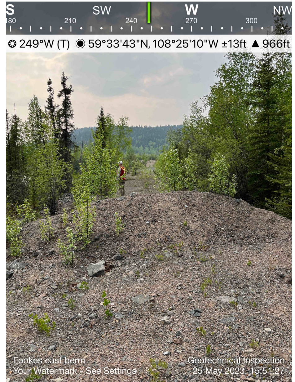
Photo C7 – View of east berm looking onto the delta. No evidence of traffic crossing the berm (May 2023).
