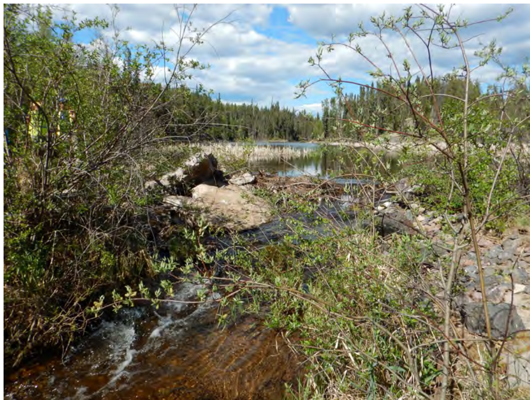
Photo A1 – Marie Reservoir Spillway looking upstream (June 2022)
