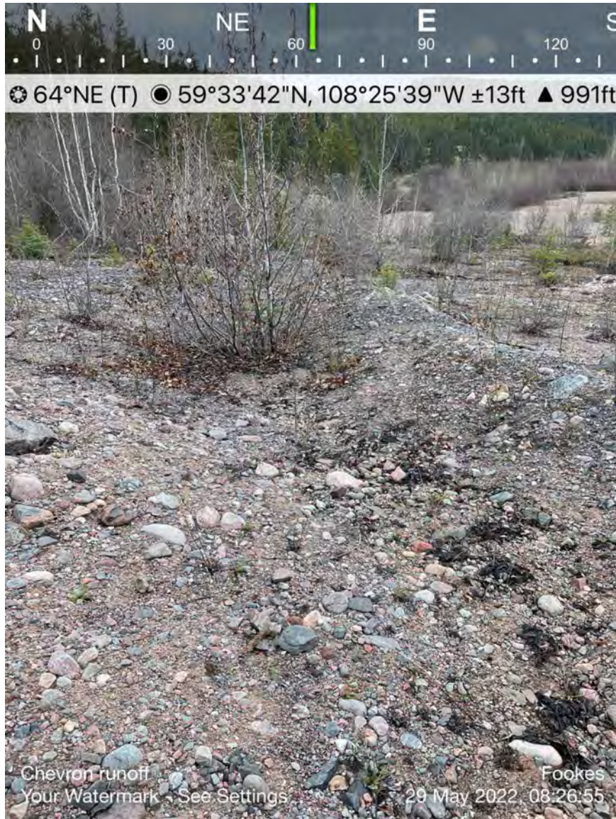
Photo C3 – Chevron run-out structure along north access road
