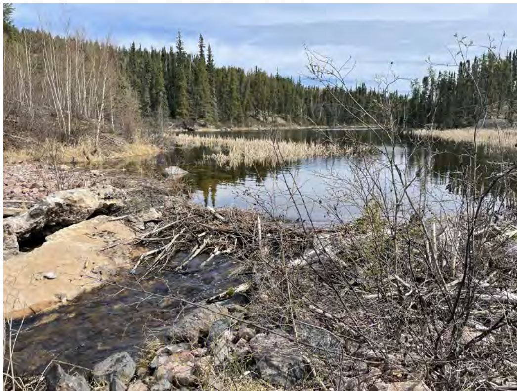
Photo A2 - Marie Reservoir Spillway inlet; beaver dam first noted in 2018
