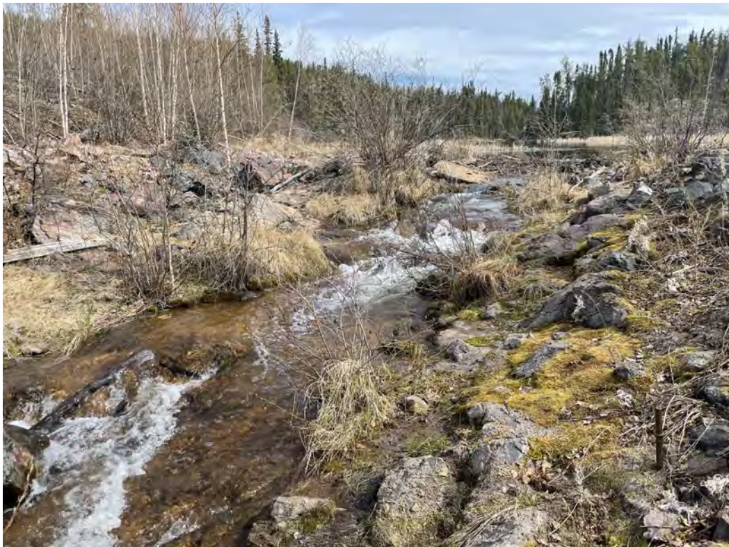
Photo A4 – Marie Reservoir Spillway looking west (May 2022)
