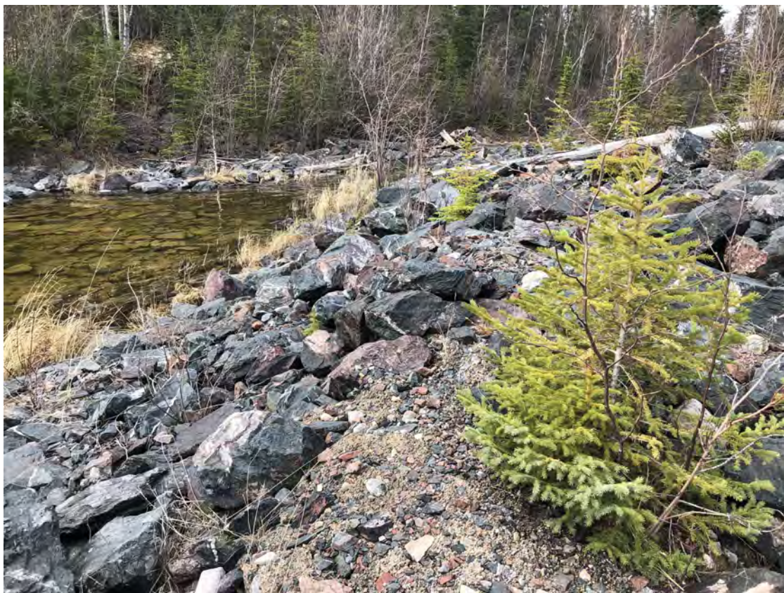
Photo B7 - Fookes Outlet— south embankment in good condition, looking west
