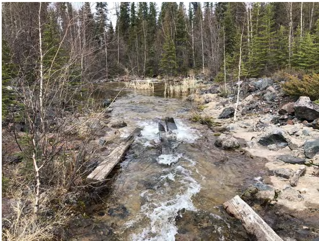
Photo B4 – Fookes Reservoir Spillway stilling basin
