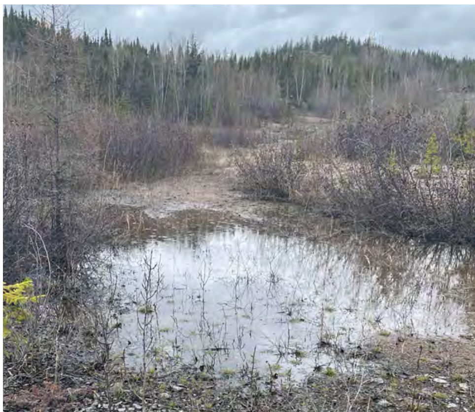
Photo C2 – ponded water on waste rock cover at bottom of hill near north access road during freshet (May 29, 2022)
