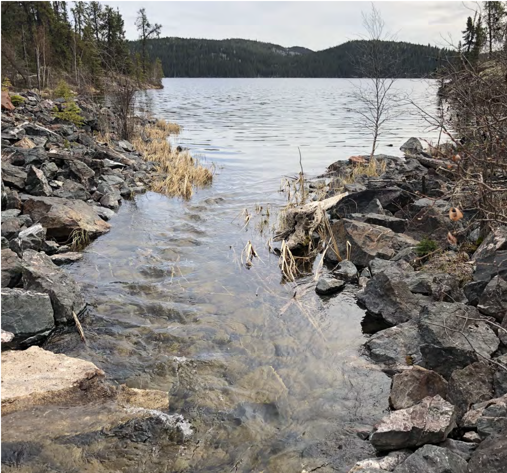
Photo B1 – Fookes Reservoir Spillway looking into Fookes Reservoir
