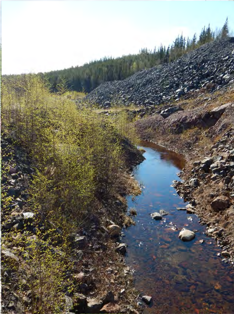
Photo E03—View near stilling basin looking upstream (May 31, 2022)
