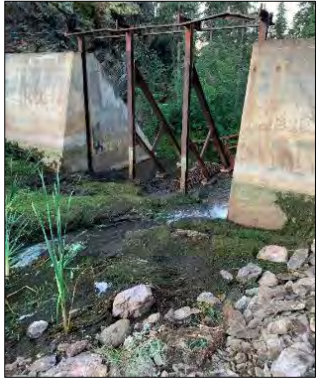
TL-7. Before and after stoplogs were moved to allow upstream to start dewatering
