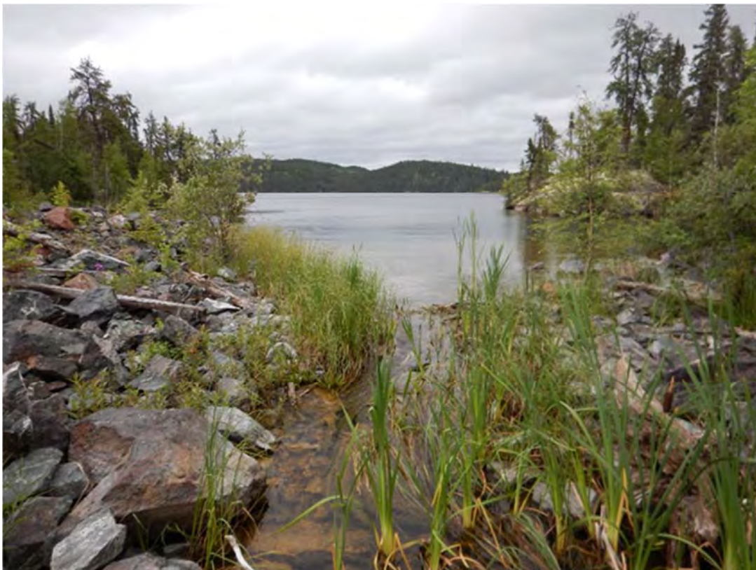
Photo B6 – Fookes Reservoir Spillway looking east
