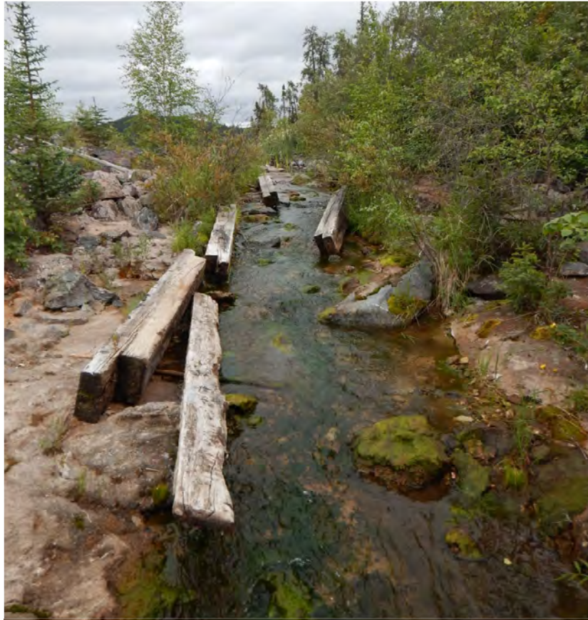
Photo B1 – Fookes Reservoir Spillway looking upstream
