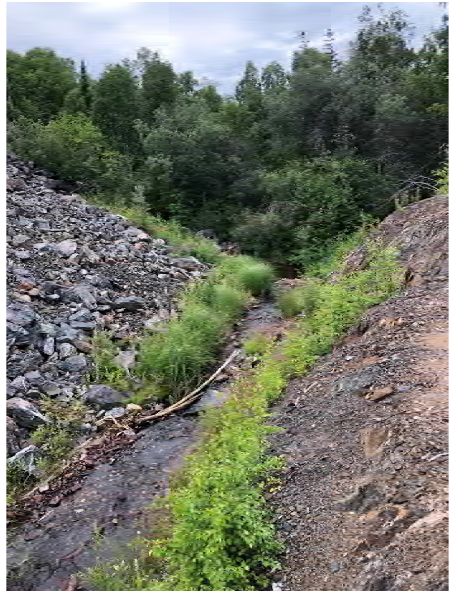
Photo E04—View near stilling basin, looking downstream at stilling basin.
