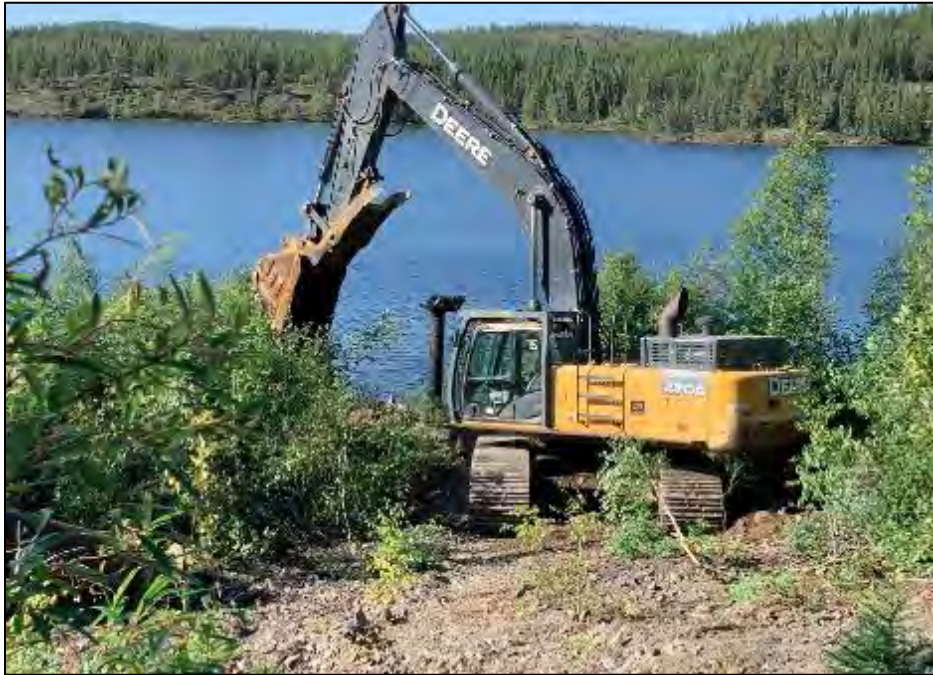
Photo 13. In-water portion of intake line has been pulled from the lake bed and is standing vertically in front of machine
