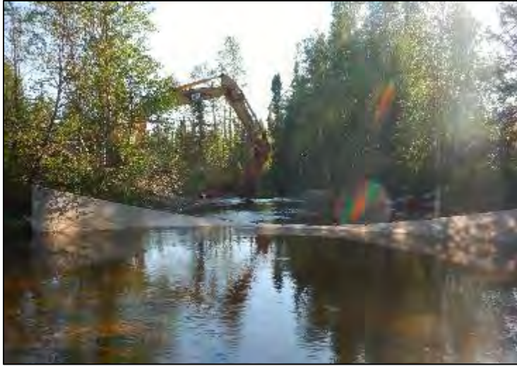
Photo 16. Net upstream of weir. Initial concrete removal to lower water levels.
