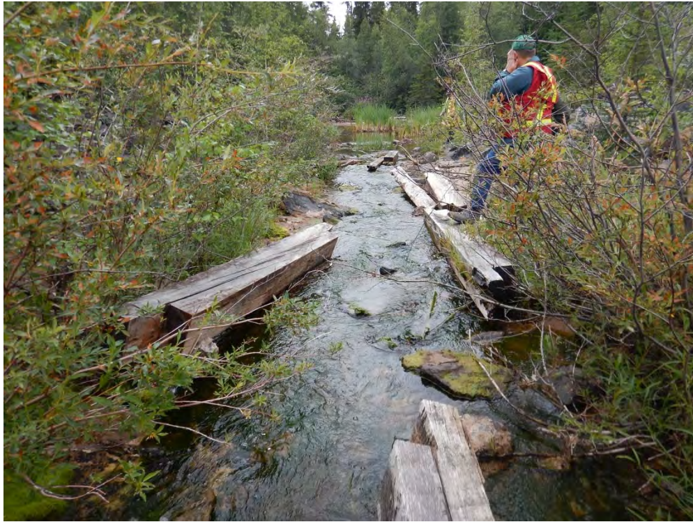
Photo B3 – Fookes Reservoir Spillway looking downstream (mid channel)
