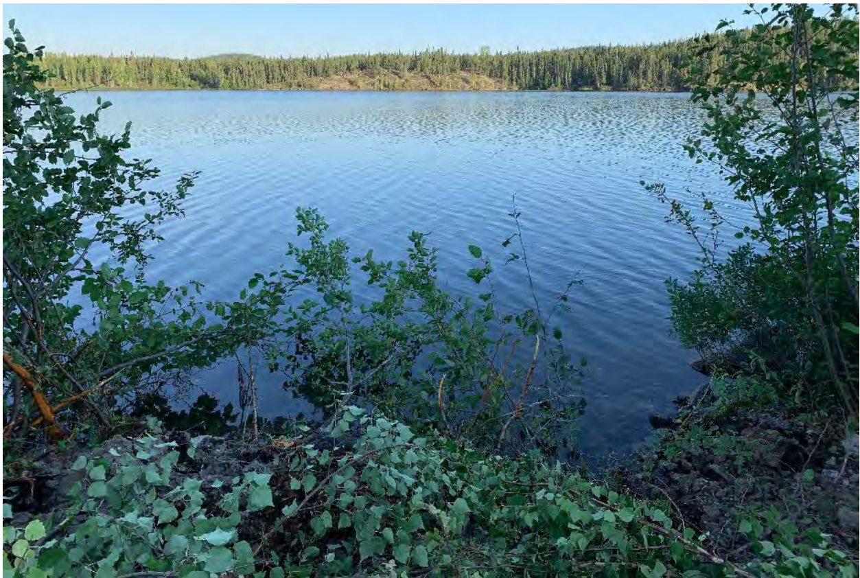
Closer view of shoreline where the pumphouse and intake line used to sit
