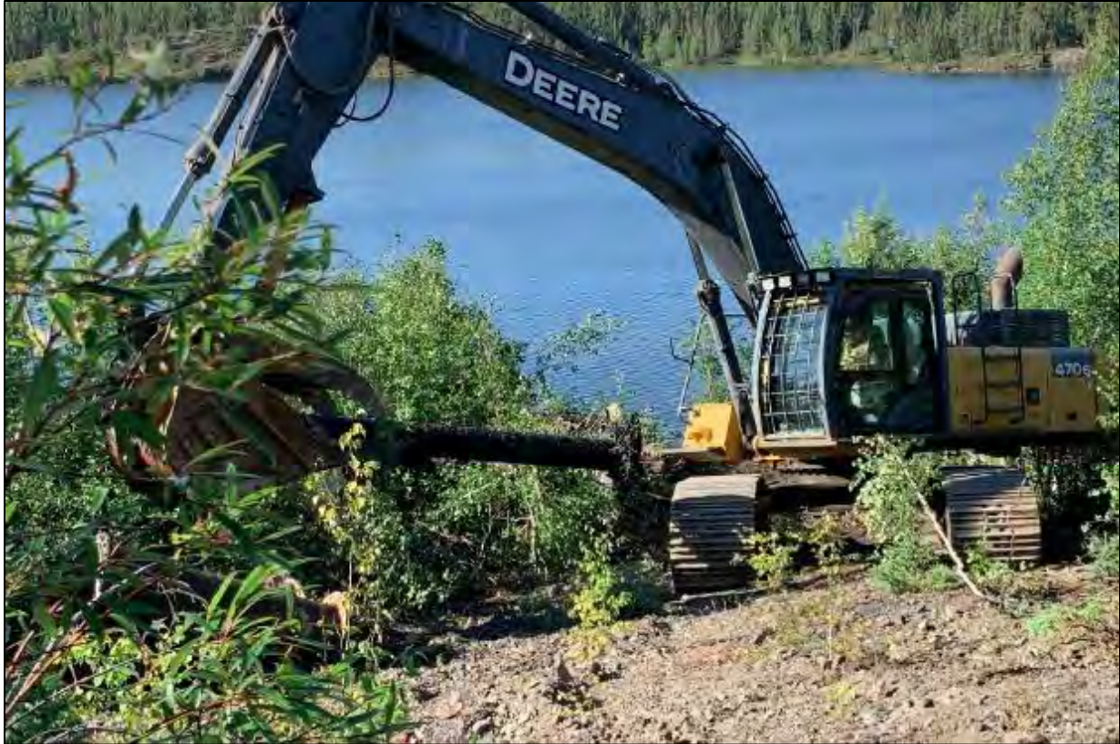
Intake from lake being moved behind excavation area.
