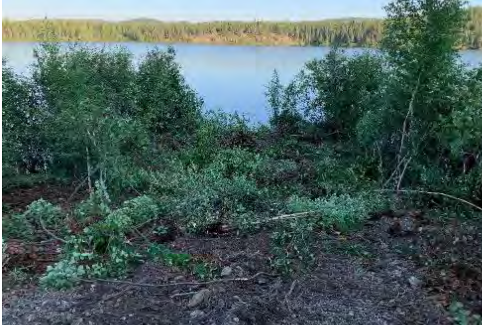
Shoreline where pumphouse was located. Slash has been placed over the backfill area
