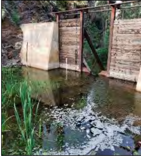
Photos 1 and 2. TL-7 prior to stoplog removal, and after water had been allowed to flow under loosened logs
