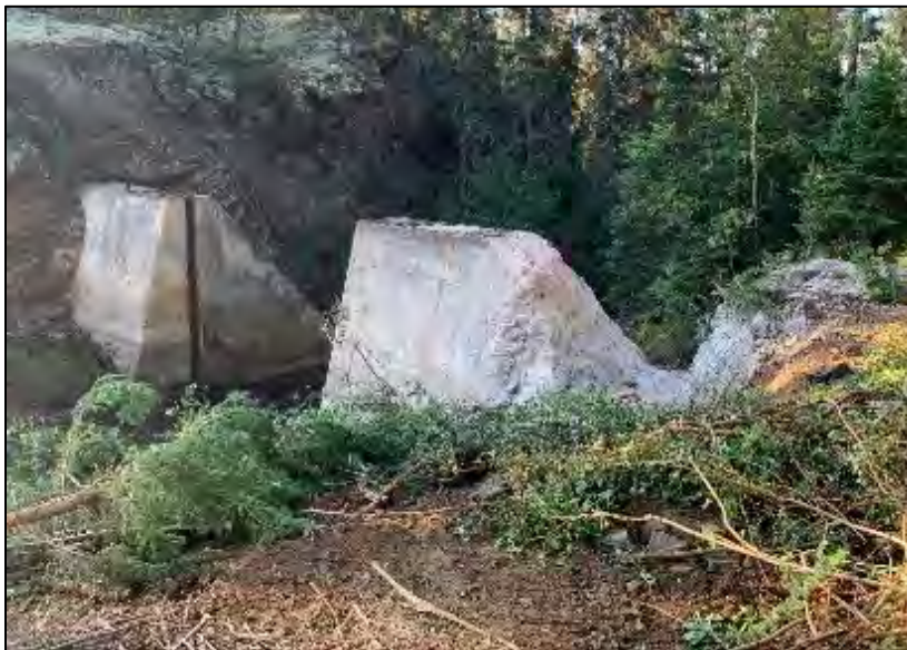
Photo 5. View from left bank, showing where concrete was chipped away
