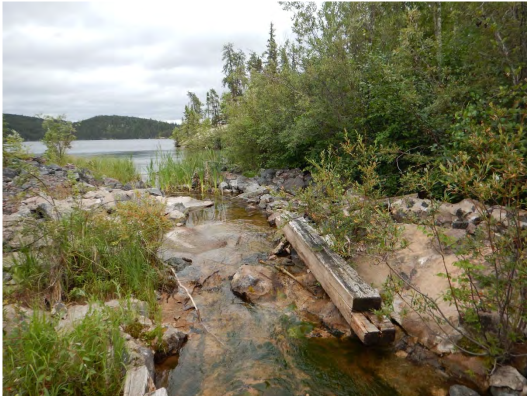
Photo B2 – Fookes Reservoir Spillway looking upstream (near mouth)
