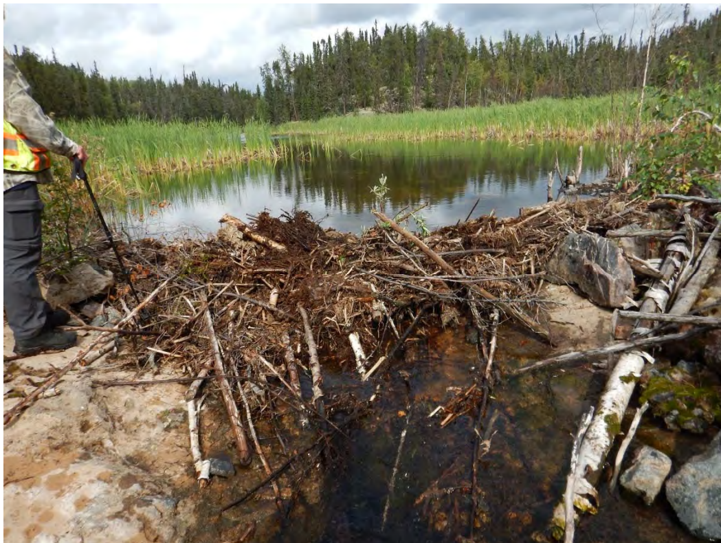
Photo A2 - Marie Reservoir Spillway inlet; beaver dam noted in 2018
