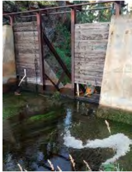
Photos 1 and 2. TL-7 prior to stoplog removal, and after water had been allowed to flow under loosened logs
