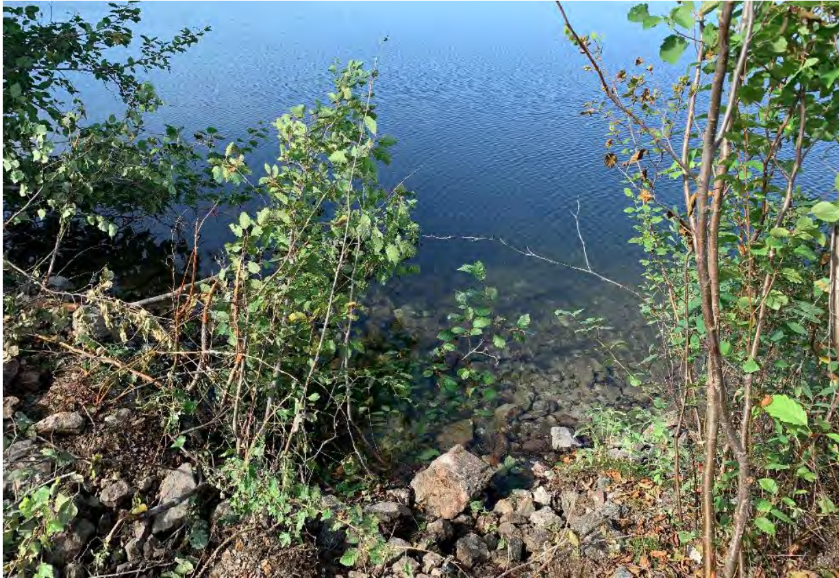
Photo 15. Location where pipeline was pulled through the shoreline of Verna Lake
