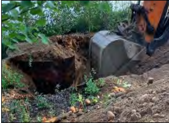
Photo 8 and 9. Further excavation behind the metal ring. It was possible to pull the ring back and avoid any excavation on the shoreline side
