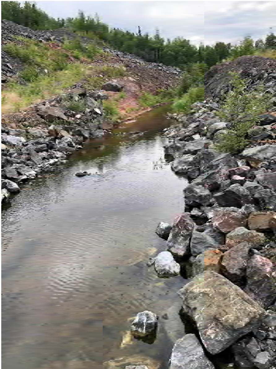
Photo E01—View from level crossing looking downstream towards Verna Lake
