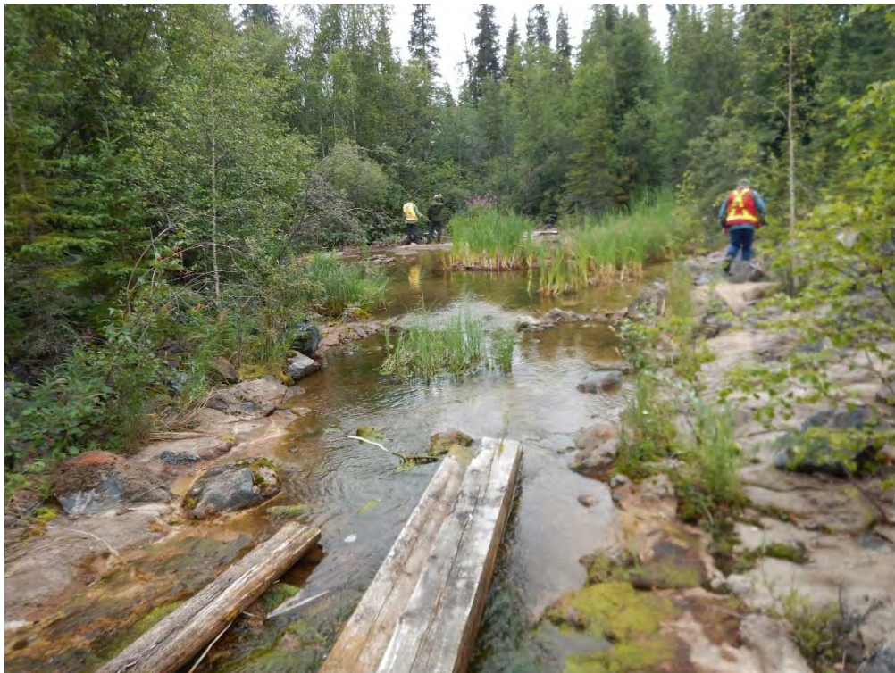
Photo B4 – Fookes Reservoir Spillway stilling basin
