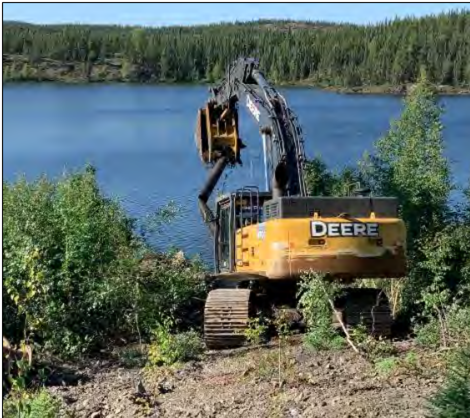
Photo 13. In-water portion of intake line has been pulled from the lake bed and is standing vertically in front of machine
