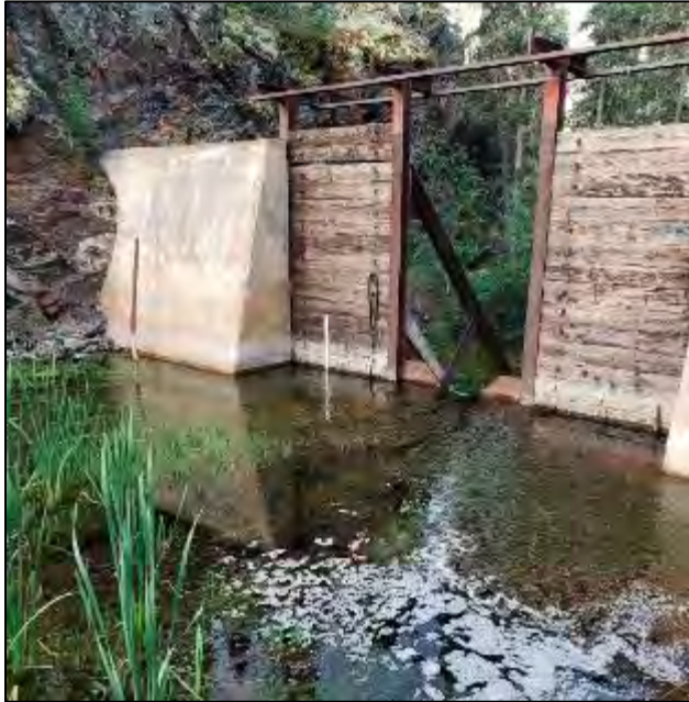
TL-7. Before and after stoplogs were moved to allow upstream to start dewatering
