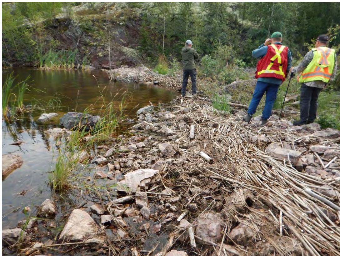
Photo A6 — Showing detritus along leading edge of embankments indicating the extent of the elevated water levels during spring 2021
