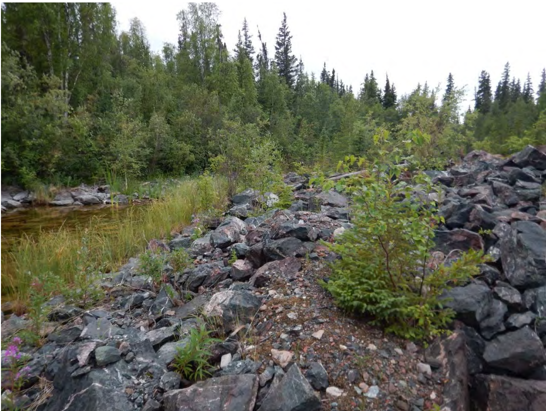
Photo B8—Fookes Outlet south embankment in good condition, looking west
