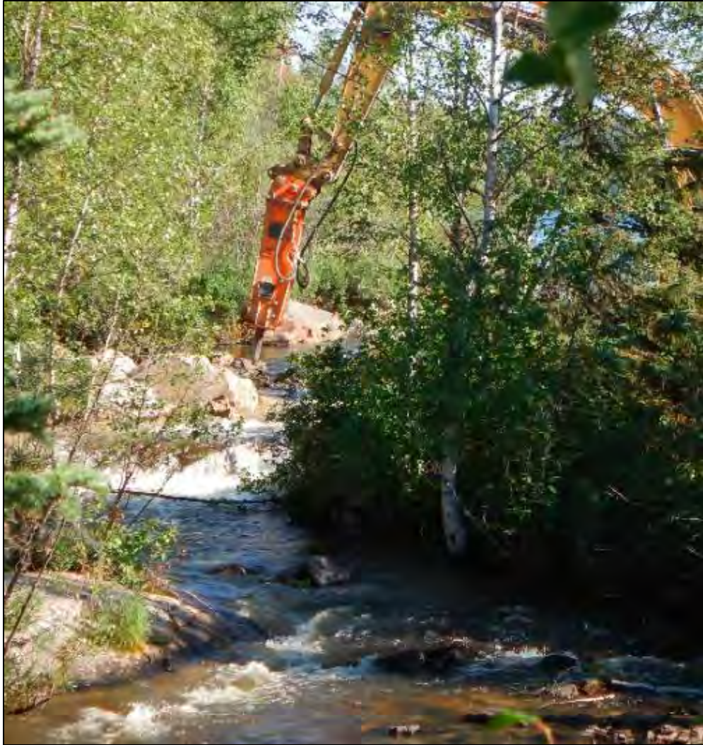
Photo 18. Concrete removal continues on Ace Creek weir
