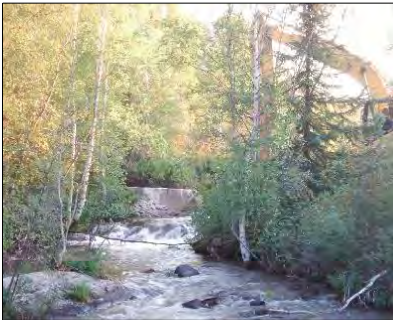
Photo 17. View looking upstream as concrete is removed from the channel.
