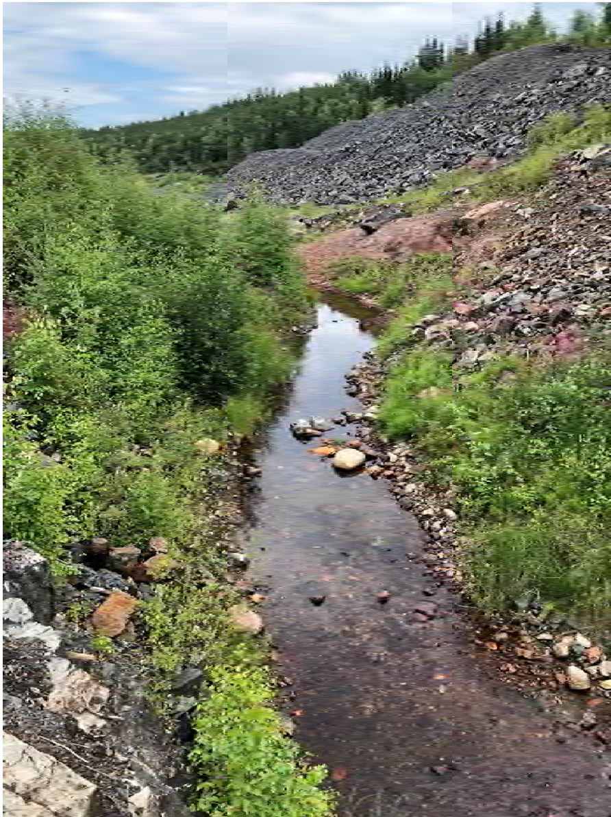
Photo E03—View near stilling basin looking upstream
