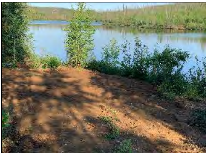
Photo 11. Looking over the excavation toward Donaldson Lake
