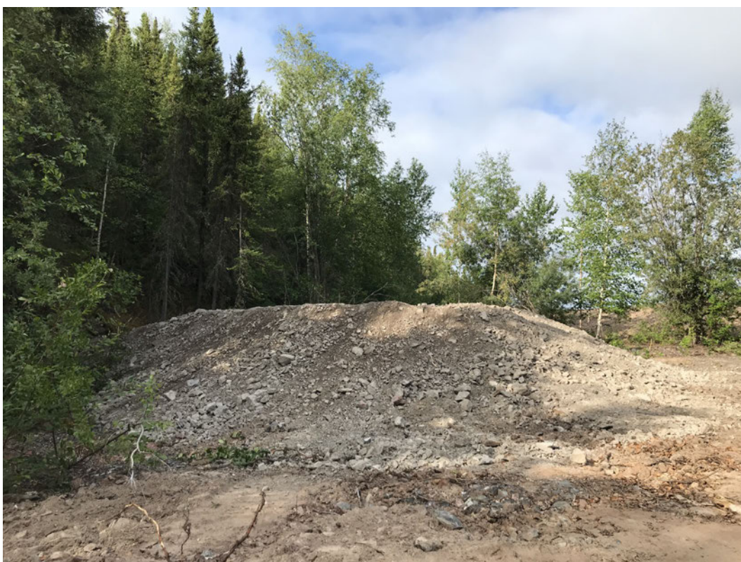
Photo D4—Stockpiled material covering the location of the 201 Stope Raise. Looking west.
