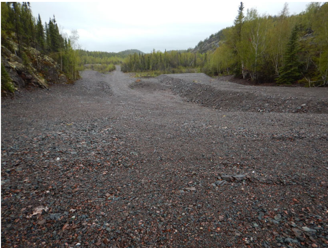
Photo D2 - View of the cover placed over Ace 201 Stope, with view to Ace 105 and 208 Stope cover on the right side of the photograph
