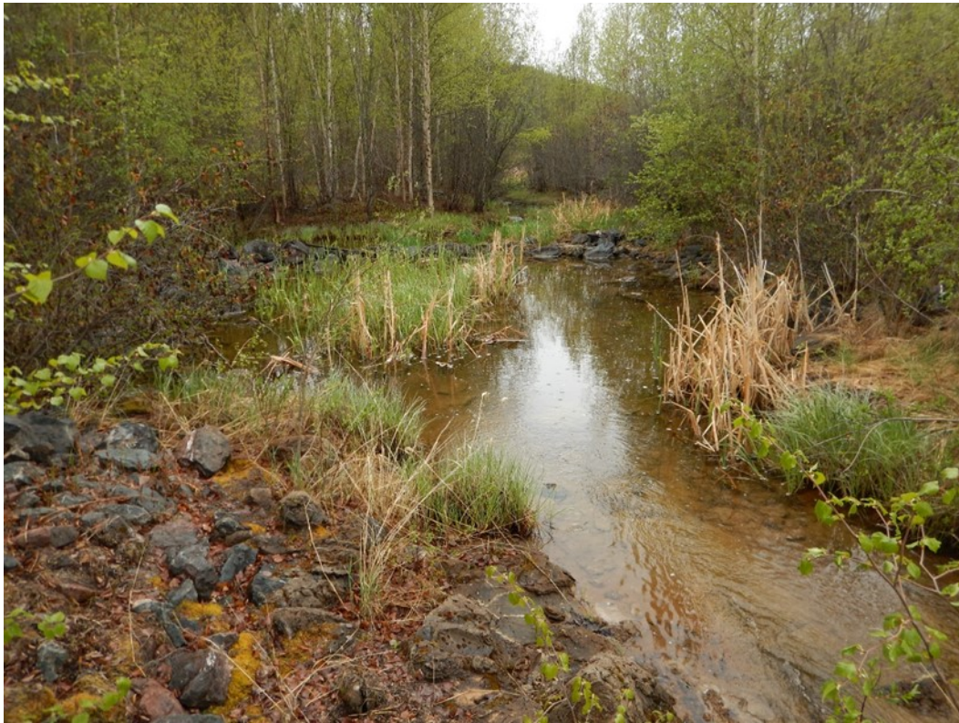
Photo A3 – Marie Reservoir Spillway (water flowing into stilling basin)
