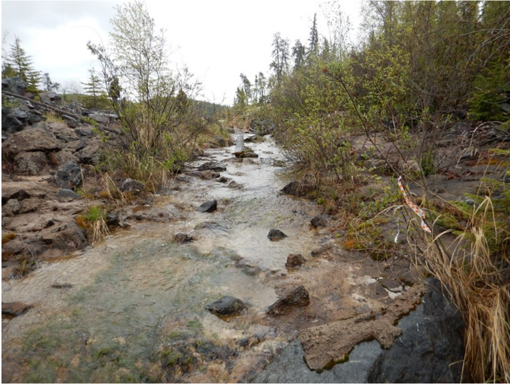
Photo B1 – Fookes Reservoir Spillway looking upstream
