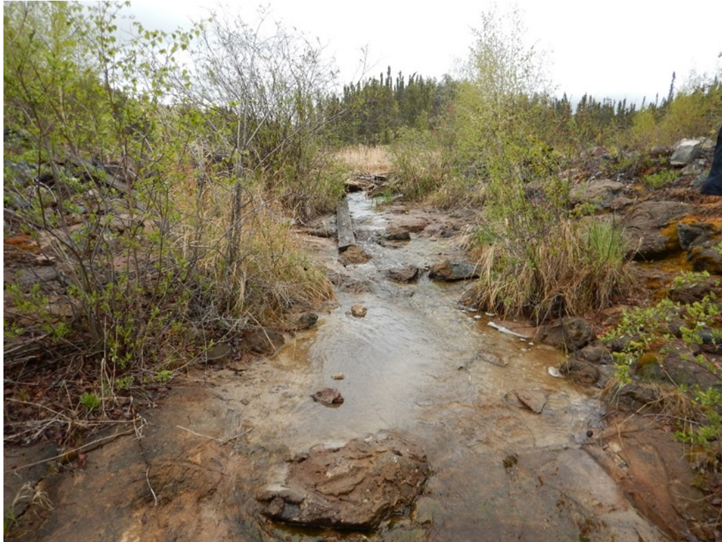
Photo A1 – Marie Reservoir Spillway looking upstream
