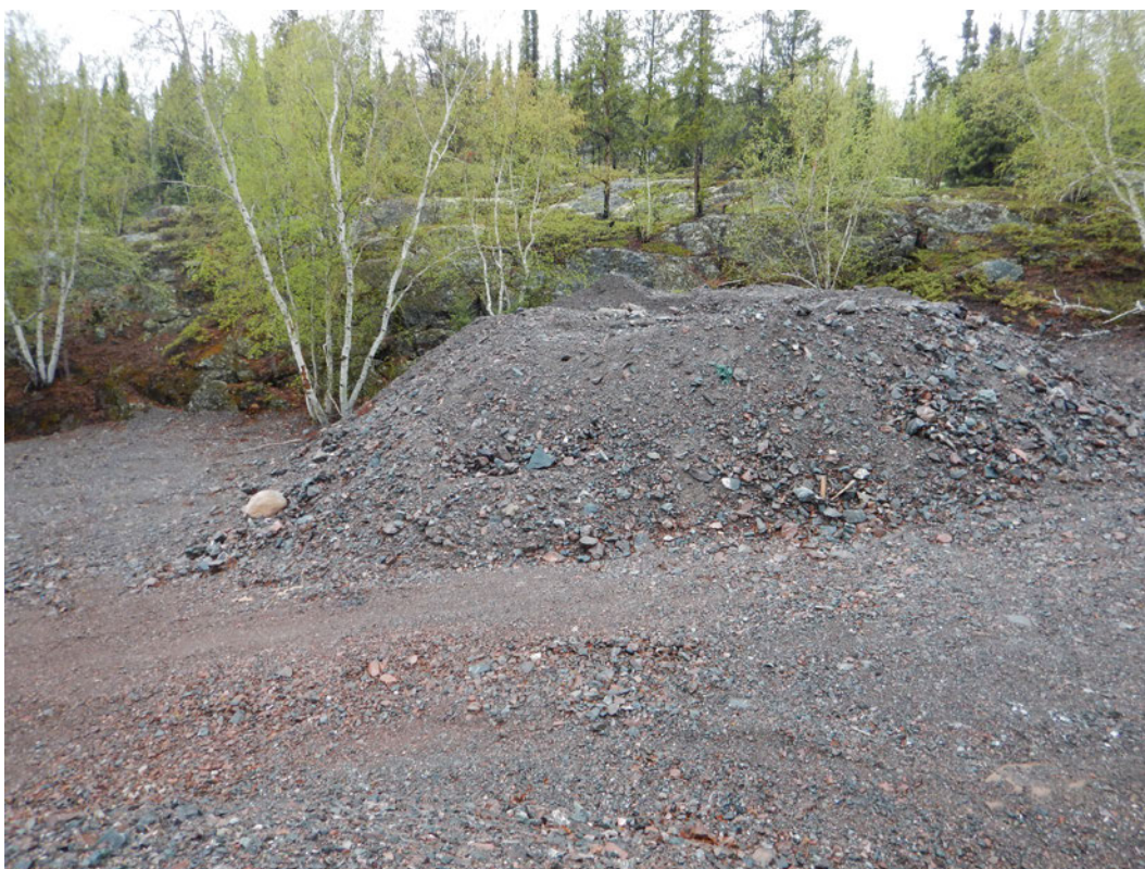
Photo D3—Stockpiled material east of Ace Crown Pillar Remediation Area, adjacent to 105#2 Stope Raise. Material to be move to location of 201 Stope Raise
