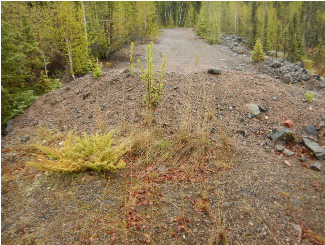
Photo C8—Protective Berm on east side of Fookes Delta (looking east)
