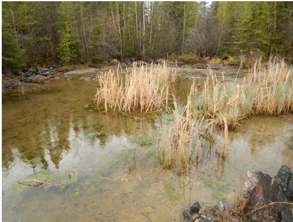
Photo B4 – Fookes Reservoir Spillway stilling basin
