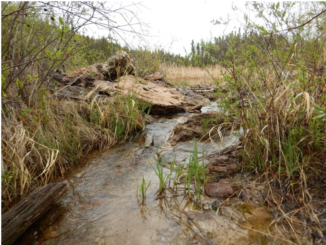
Photo A4 – Displaced grout intruded rip rap at the entrance to the spillway
