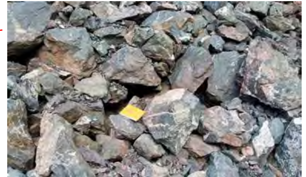
Photo 11 – Example of a typical waste rock void on crest and slopes.
