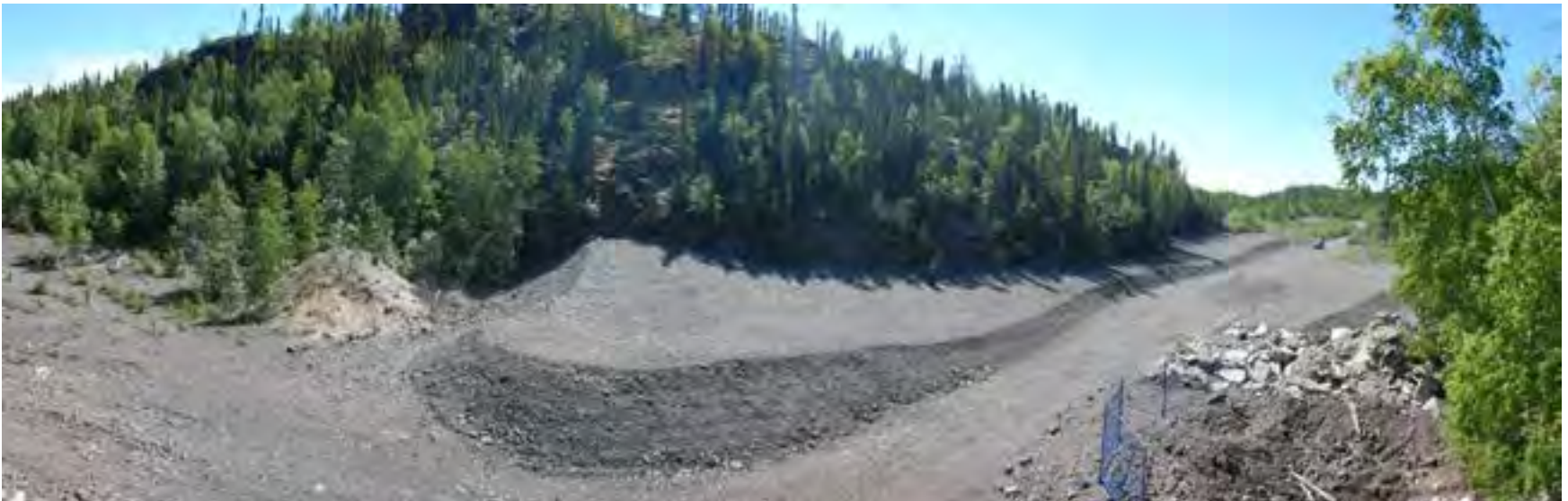
Photo D6 - Panorama photo looking south-west showing Stope 103/201 crown pillar cover on the left and Stop 208 crown pillar cover on the right. Vent Raise 105 is in the foreground (on the right) and has since been remediated.
