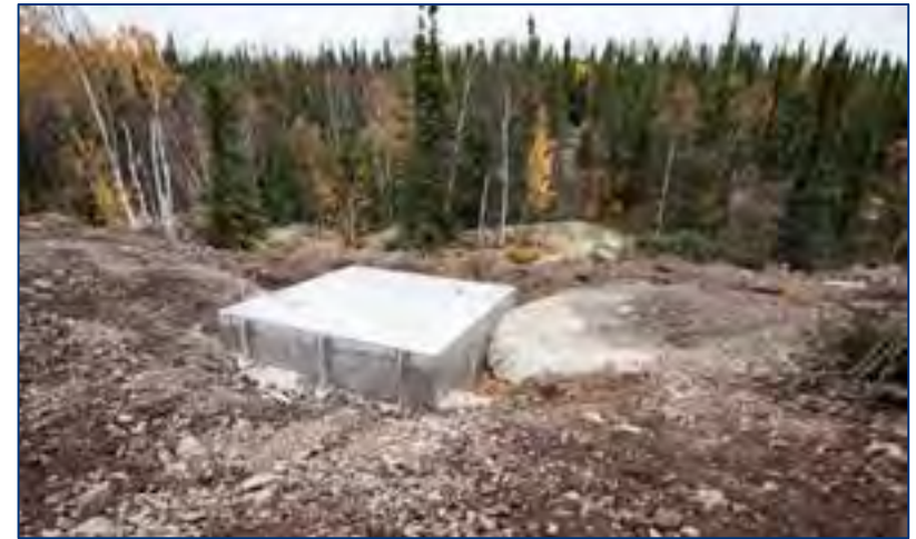
Completed cap at Ace 130 Raise
